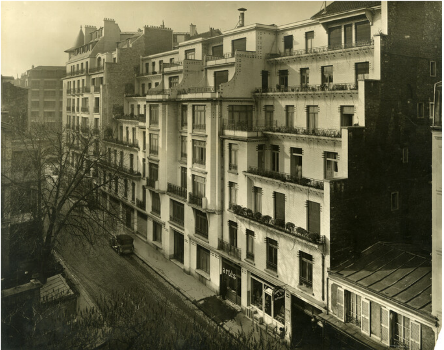
Henri Sauvage and Charles Sarazin, terraced residential building clad in glazed white ceramic tiles, 26–28 rue Vavin, Paris, 1912–1913. Photograph by Chevojon. Image © Fonds Sauvage, SIAF/Cité de l'architecture et du patrimoine/Archives d'architecture du XXe siècle.
