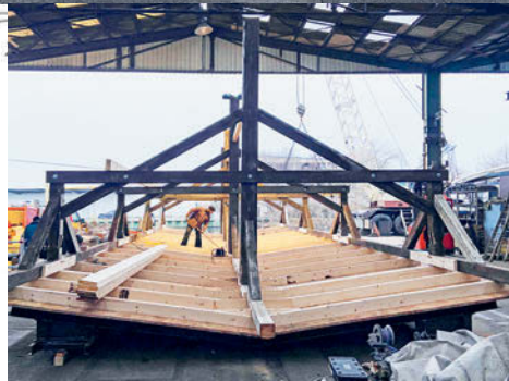
The roof truss after dismantling
